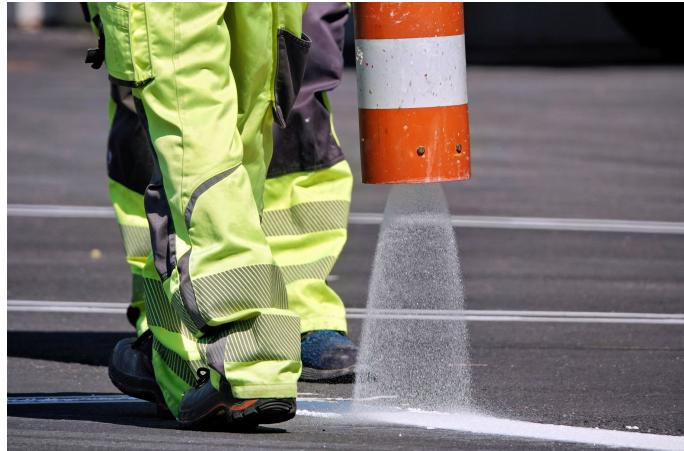
In addition to drop-on applications, SWARCO SOLIDPLUS retroreflective glass beads can also be integrated directly into the marking material during the production of thermoplastics, cold plastics, or comparable road marking systems.
